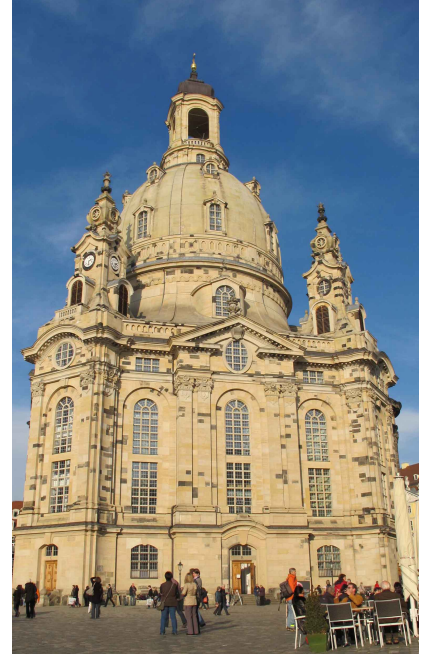
Dresden Frauenkirche, first built between 1726 - 1743, rebuilt in 1990
